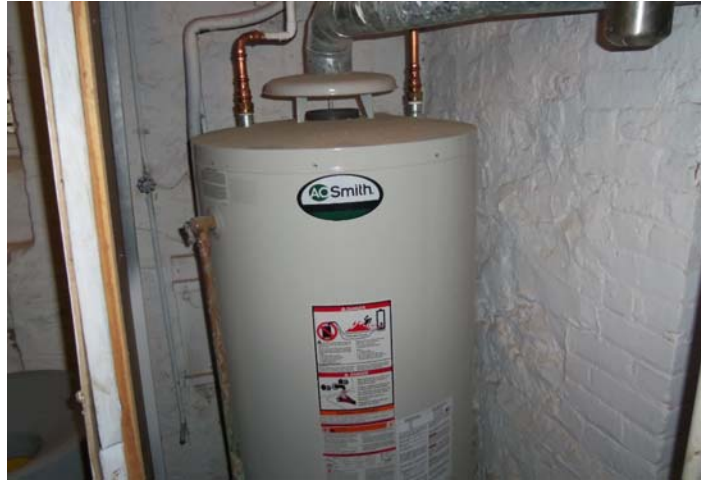
4: Domestic hot water heater
