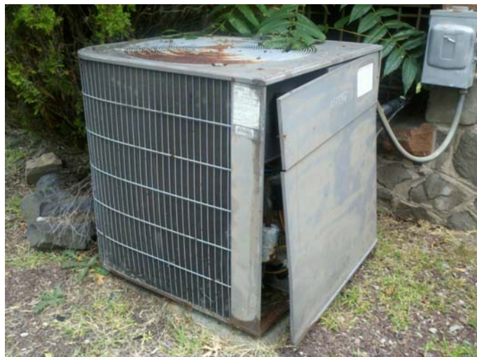
3: Inoperative condensing unit
