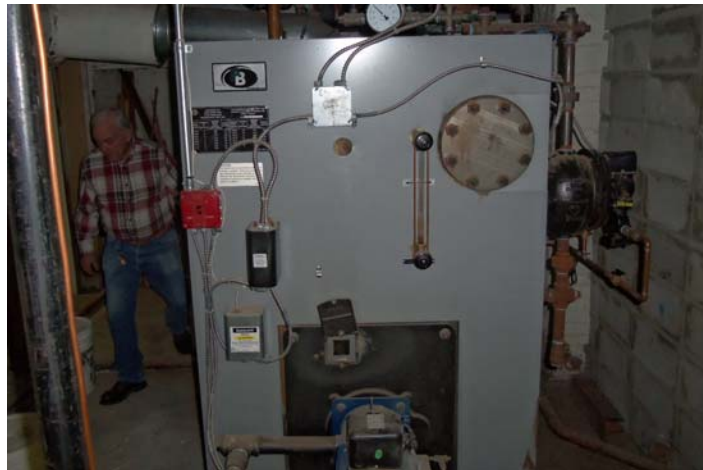
2: Steam boiler in basement
